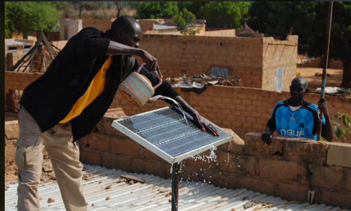
Photovoltaic devices installed to charge solar lamps in African schools
